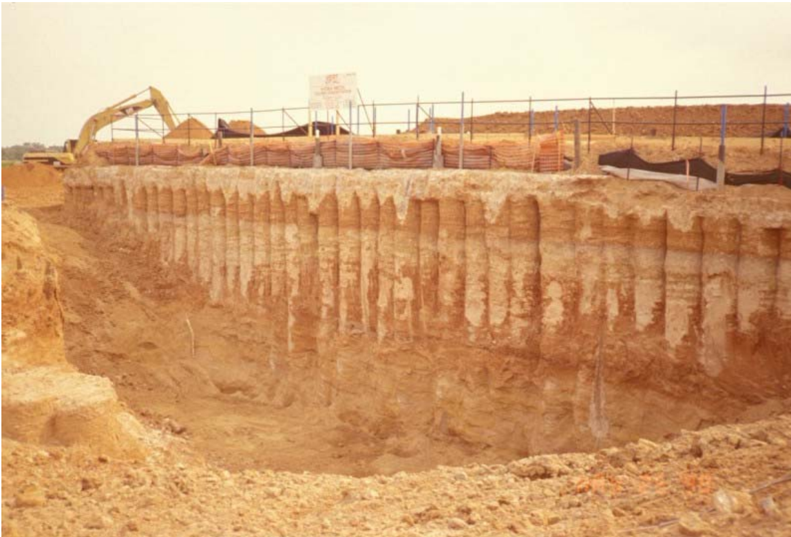
Figure 4 – 8. Completed VERT Wall (After Briaud et al., 2000)
