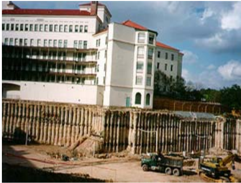
Figure 2 – 5. Hermann Hospital, Houston, TX Excavation (Picture from Schnabel Foundation Company, www.schnabel.com )
